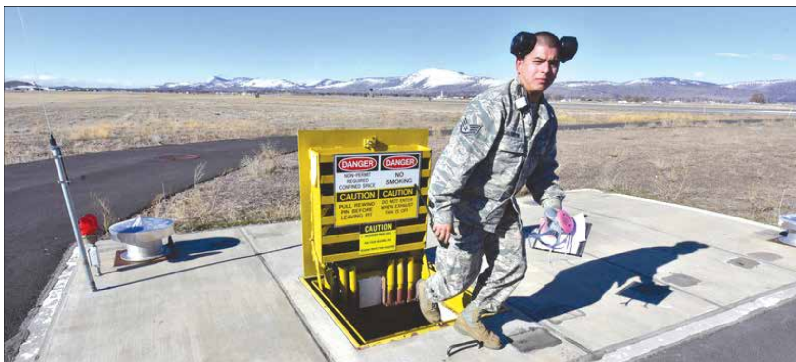
U.S. Air Force Staff Sgt. Eduardo Calderon, the sole arresting system certifier at the 173rd Fighter Wing in Klamath Falls, Oregon, emerges from an underground room after inspecting the emergency arresting system following a test of the system at Kingsley Field in Klamath Falls, Oregon, March 7, 2019. It is necessary to construct the rooms underground because the airfield is required to be flat and without obstruction, particularly this close to the active runway. (U.S. Air National Guard photo by Tech. Sgt. Jefferson Thompson)
